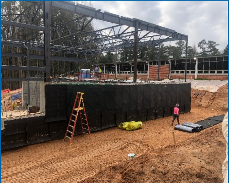
West Gym Foundation Backfill & Waterproofing
